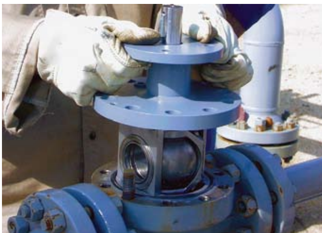
FIG. 2 The cartridge may be removed by unbolting the bonnet fasteners and lifting the cartridge from the valve body.
